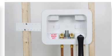
RIGHT DRAIN, BOX MOUNTED ON RIGHT STUD
