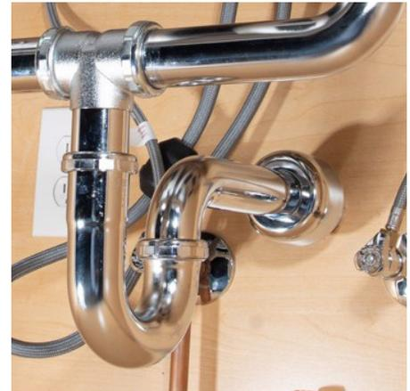
**3** Insert the wall tube into the waste connector and hand tighten. If using a 1-1/4 in. wall tube with a 1-1/2 in. waste connector, use a reducing washer to make the transition.
